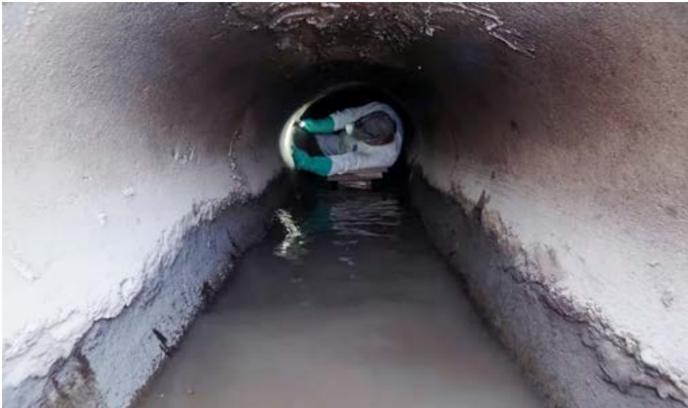
↑ The working space is tight for an FID staff member making repairs inside a water conveyance pipeline.
