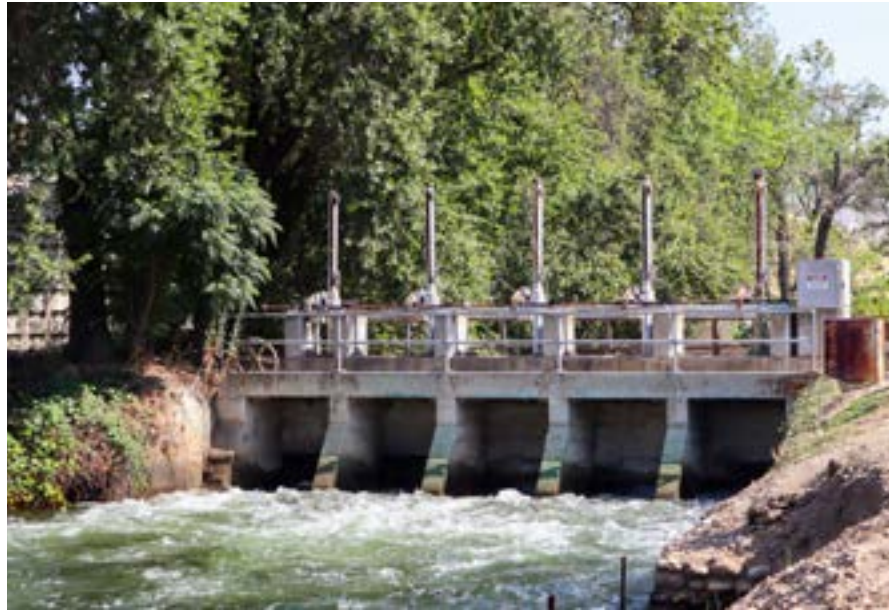
↑ At Gould Weir two miles upstream from Fresno Weir, this headgate structure diverts FID water into the Gould and Enterprise canals to serve northern and eastern portions of the District.
