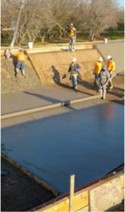
↑ Concrete lining is installed along an FID canal section.
