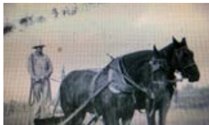
↑ Maintenance work is performed on an early-day Fresno Irrigation District facility by an FID worker operating a horse-drawn Fresno scraper. Invented in Fresno County, such scrapers were used until mechanized bulldozers were developed.
