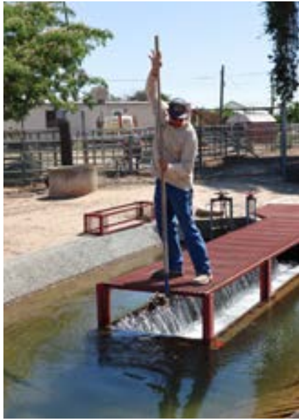
↑ Debris being removed from one of FID's long-crested weirs used in regulating canal deliveries.
