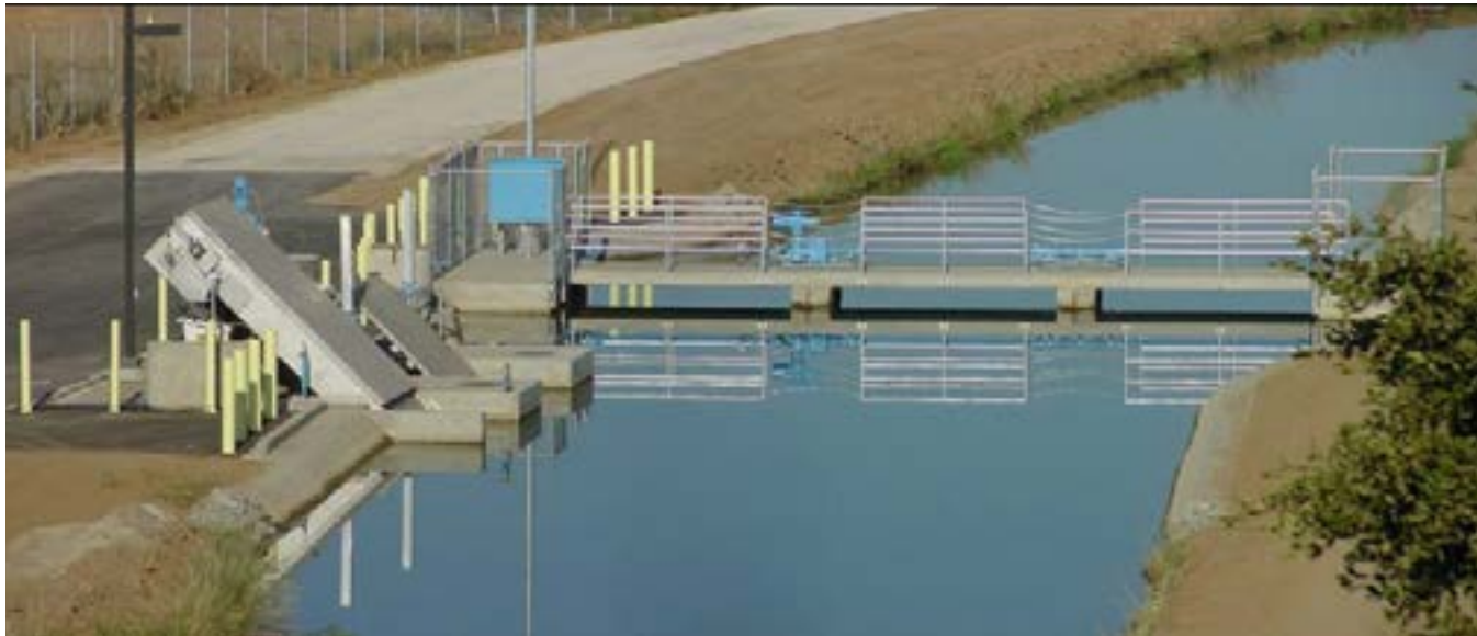
↑ FID's Enterprise Canal's turnout to the City of Clovis' Surface Water Treatment Plant, a state-of-the-art facility. It treats raw surface water to drinking water standards for Clovis residents. Control gates regulate the City's diversions. Trash racks remove large debris. FID has been conveying water to this plant since it came online in 2004.
