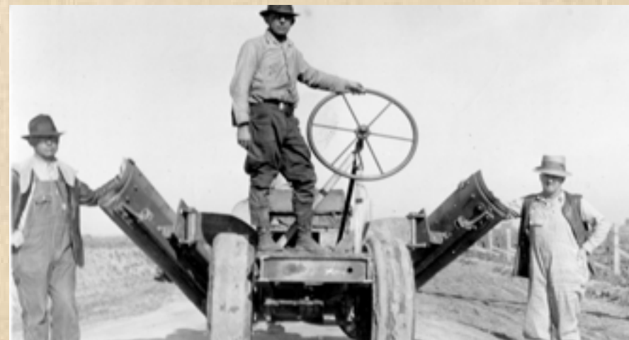
← In later decades, development of sloper devices for cleaning canal banks proved to be a significant Fresno Irrigation District maintenance aid.
