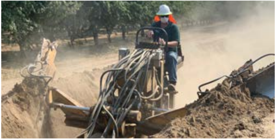
↑ FID worker operating the sloper, used in re-sloping the canal banks.
