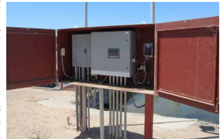
↑ SCADA equipment stands alongside an FID canal as part of a District-wide control system including computers, data communications networking and related conveniences to process water system operational orders.
